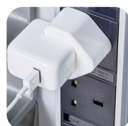
Device adapters plug into 2x10-way powerstrips.
